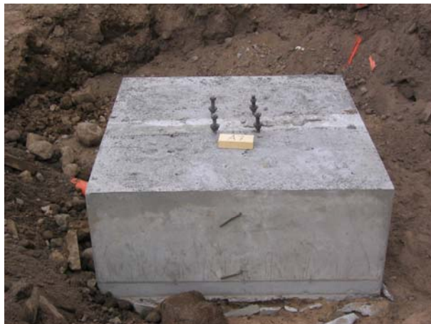
Figure 29 Concrete slab casted directly on the block of 9 columns.
