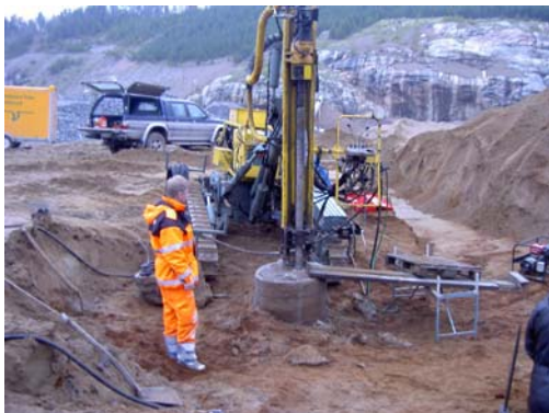
Figure 9 Core sampling performed in MDM-columns.
