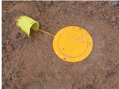
Figure 13 Pressure cells installed above column, on a cushion of sand (Soil Instruments Ltd).
