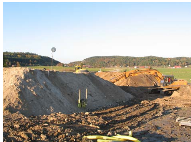
Figure 11 Construction of 3 m high test embankments.
