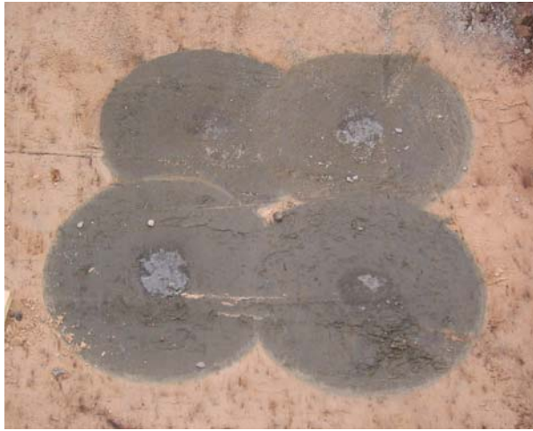
Figure 28 Block of columns excavated down to cut-off level directly after installation.
