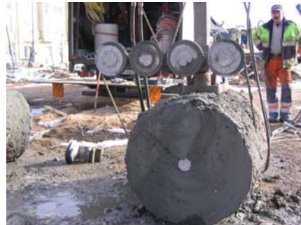
Figure 25 Cutting of extracted columns using a wire saw. The GEWI-bar is visual in the middle.
