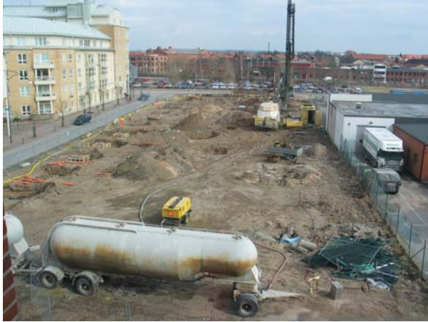
Figure 22 View of the construction site at Gamletull, in Halmstad.
