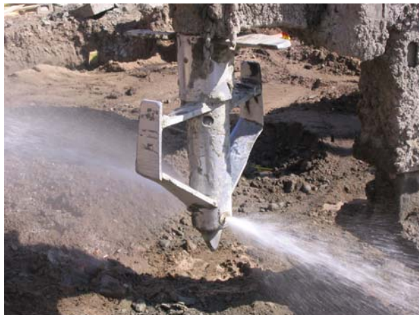
Figure 2 Example of mixing tool used at the Gamletull jobsite in Halmstad. Binder outlet and valves for water are shown.
