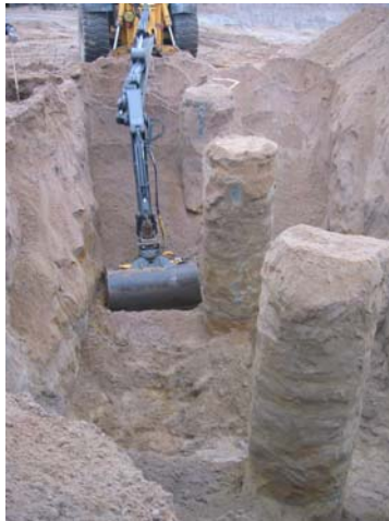
Figure 8 Columns installed with 450 kg/m 3 cement in semi-dry sand.
