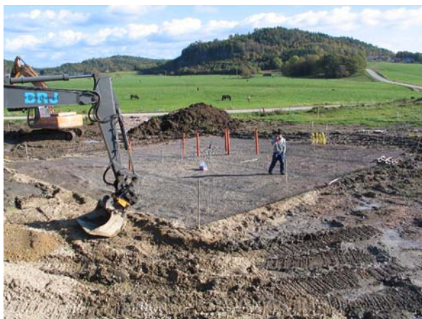
Figure 12 Installation of load transfer platform.
