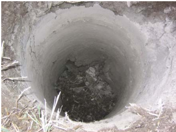
Figure 5 Crater experienced during installation of Dry Mix column.
