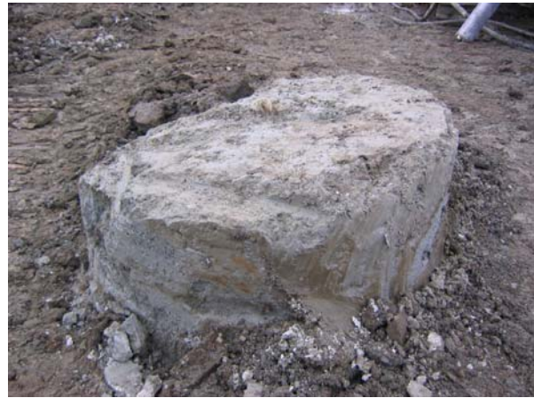
Figure 6 MDM column performed through the dry crust. Excavation has been conducted for the upper 0.5 meters.
