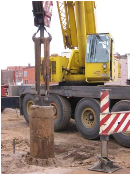
Figure 23 Extraction of whole columns.
